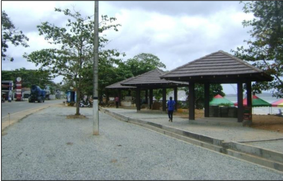
Picture 31: Constructed Fish Stalls - Stage I – Beach Development Project
