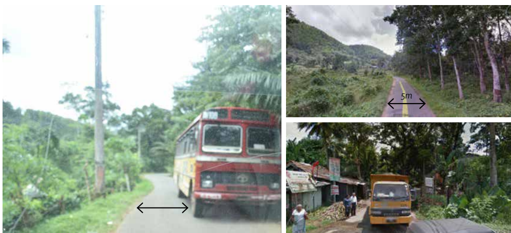
Image 5.2 : Condition of Existing Narrow Road in the Area
