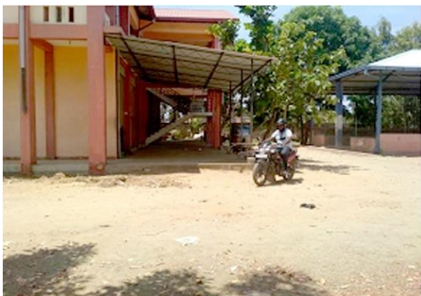
Figure: Existing Public Market building
