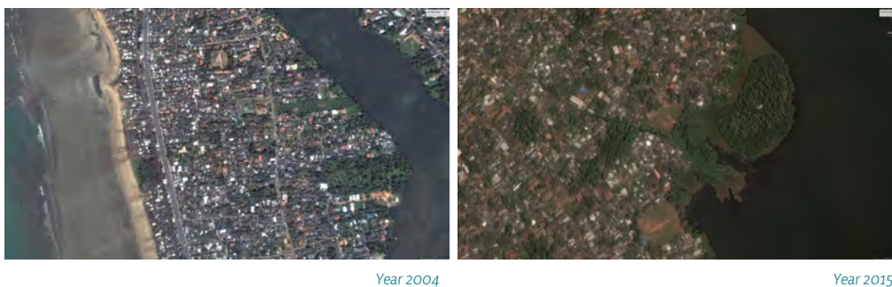
Figure 5.2 : Unauthorized Reclamation of Lands Surrounding Area of the Maduru Doowa (Island) Source : Google Earth, 2018
