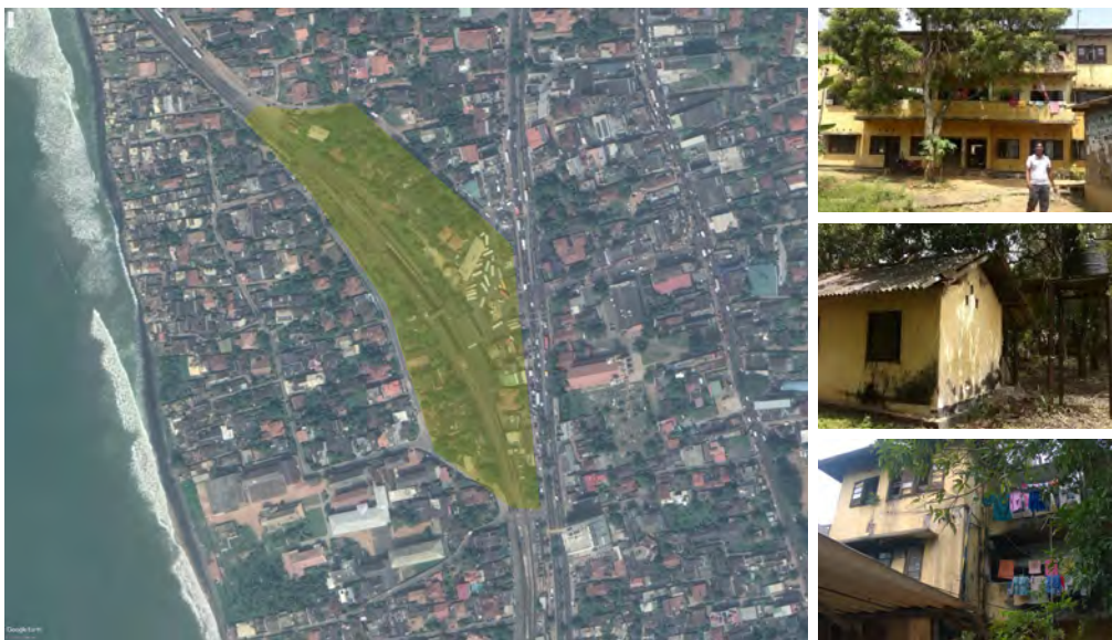
Figure 3.4 : The Land owned by the Department of Railway Image Courtesy : Urban Development Authority, 2017
