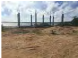
Existing Building 'A' (Only foundation structure is remained at the existing situation)
