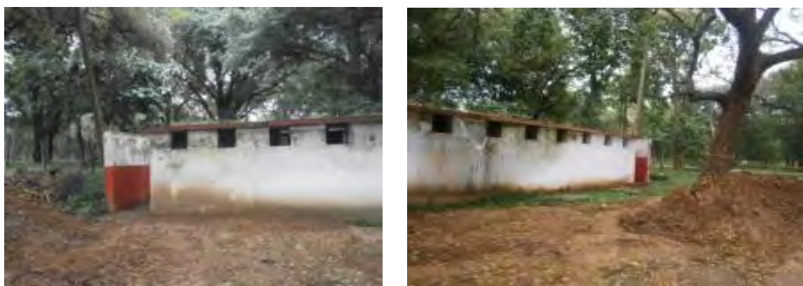
Figure 5.21. Public Toilet Rooms in Kataragama
