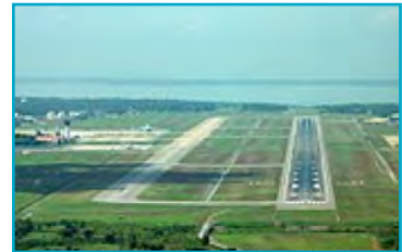
Figure No 5.3.1.A.3 Palawiya Air Port
