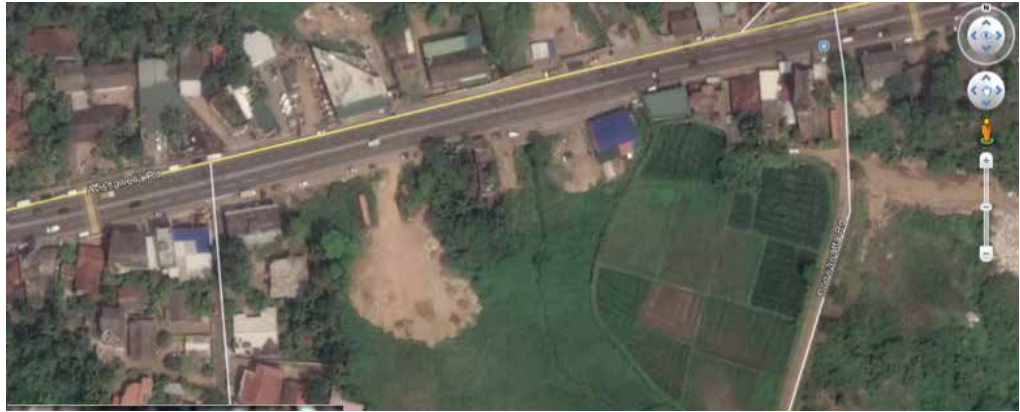
Figure 5.4 : Unauthorised Landfilling along High Level road Source : Google Earth
