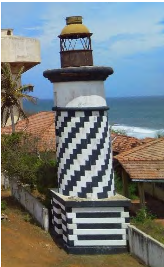
Figure 5-6: Ancient Light House- Towerhill
