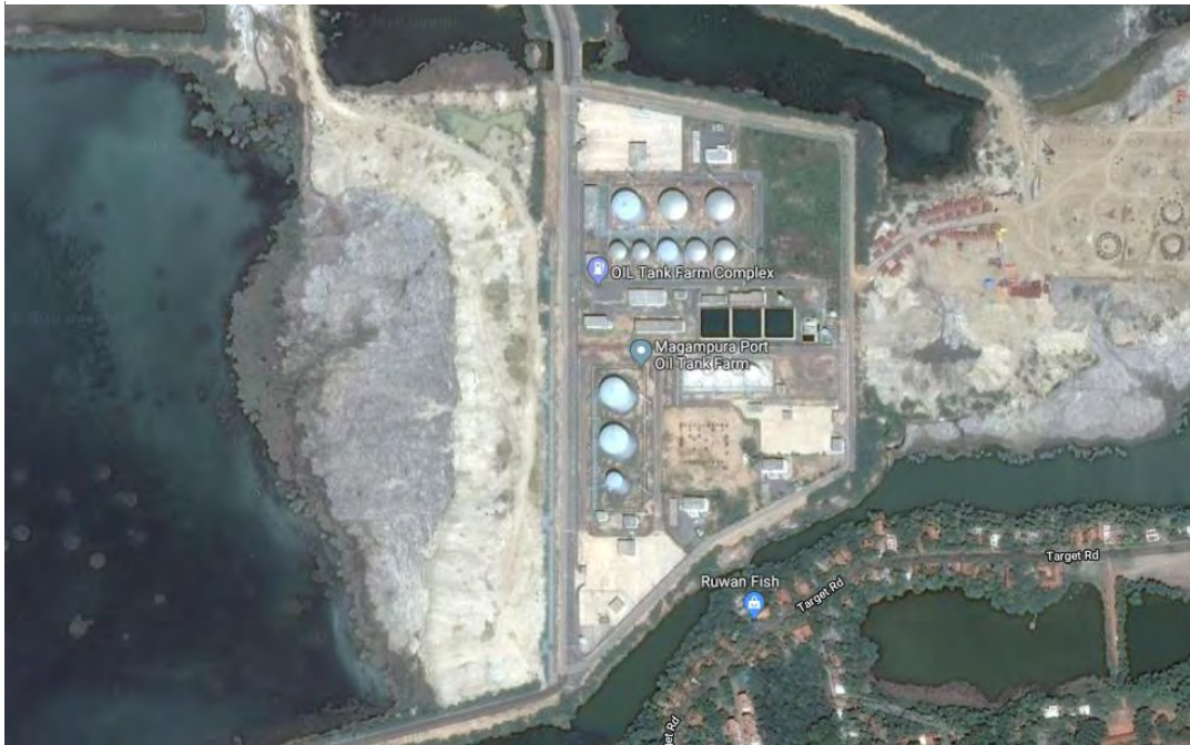
Figure 5-19 : Oil & Gas Refining Yard
