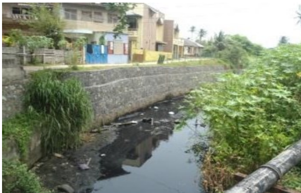
Figure 5.1-22: Kepu Ela, Mahamodara Lake & Old Dutch Canal
