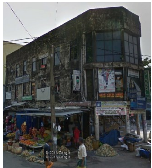
Dilapidated building at Sea Street
