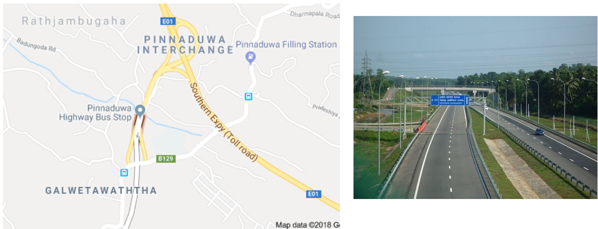
Figure 5.1-35: Pinnaduwa Interchange of Southern Expressway
