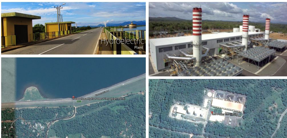
Figure 5.11 : Udawalawa Hydro Power plant
