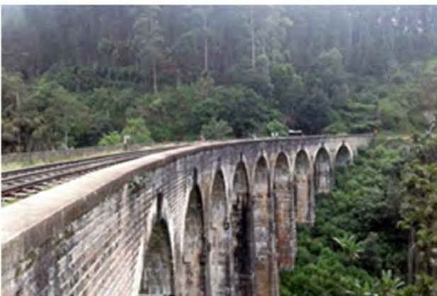
Arches Bridge in Demodara
