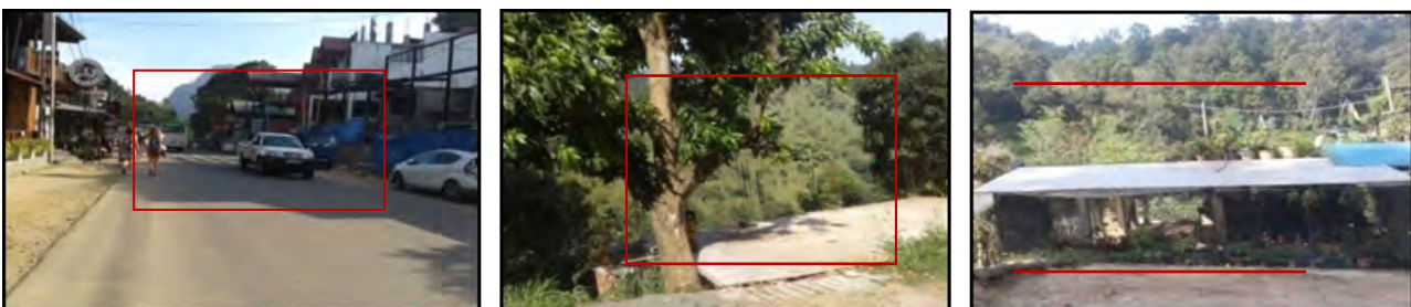
Figure No 5.4: Unauthorized constructions in the Ella Town
