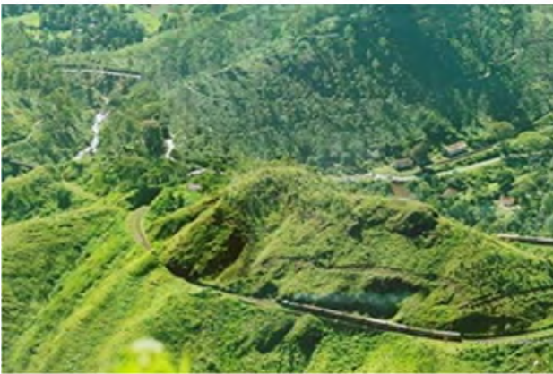
Demodara Rail Track – Engineering Masterpiece
