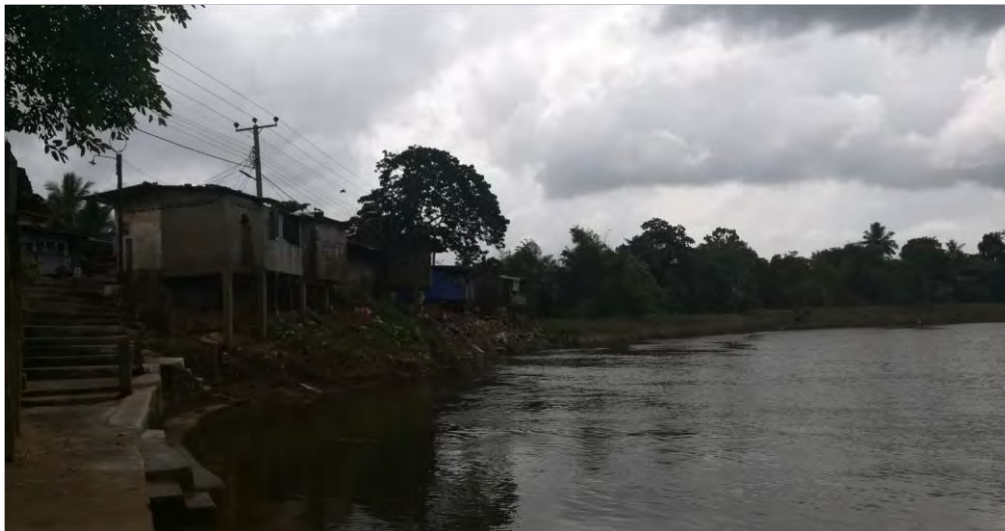
Figure 5.21 Kelani River Reservation Encroachments - Malwana
