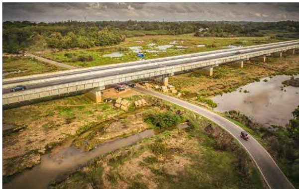
Figure 2. 6 Outer Circular Highway
