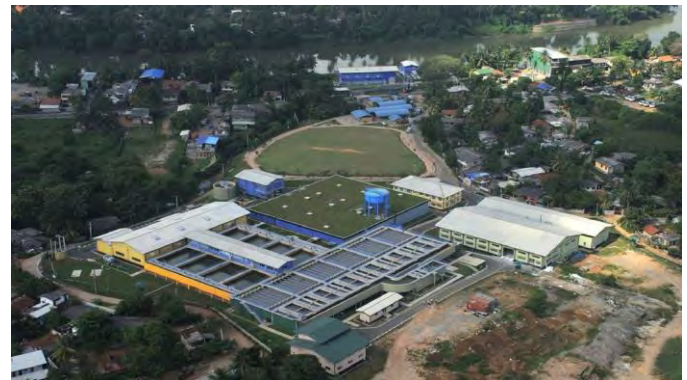
Figure 2. 7 Kelani River Right Bank Water Treatment Plant
