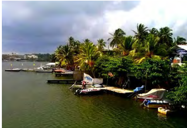
Figure 3.7: Unauthorized constructions in the Benthara river reservation | Source: Photography by Beruwala planning team, Kalutara District Office – 2018
