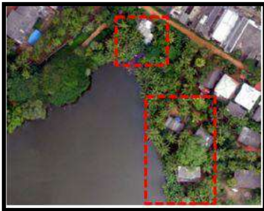
Figure 5. 26 Unauthorised construction in spill canal of Nuwara Wewa
