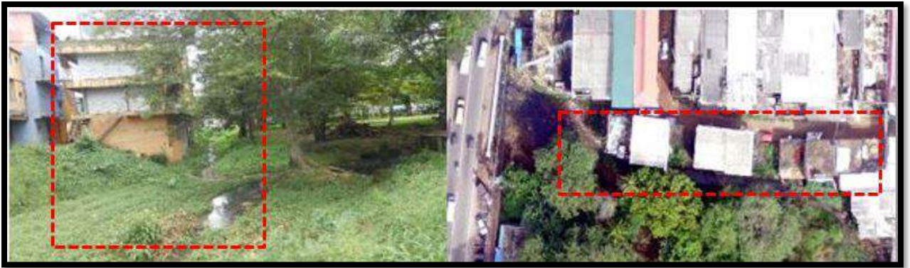
Figure 5. 24 Unauthorised construction in reservation of Kadapanaha Wewa
