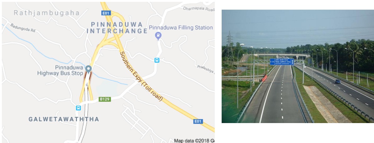
Figure 5.1-8: Pinnaduwa Interchange of Southern Expressway
