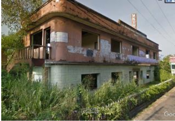
Degraded buildings at Pettigalawatta
