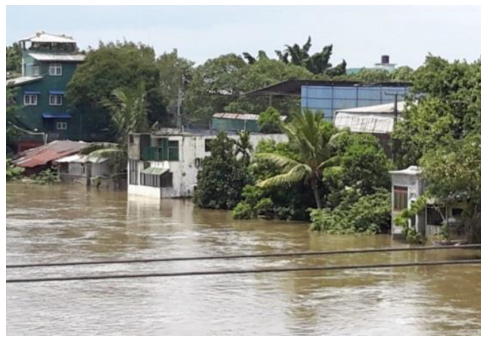
Figure 121: Partially inundated houses on left bank of Kelani River on 20th May 2016 (approx. 2.2m flood water level) | Source: Flood Hazard Assessment & Hydraulic Modelling; deltares, adpc & cecb, 2017
