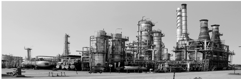
Figure 45: Kolonnawa Petroleum Refinery Image Courtesy: ceypetco.gov.lk
