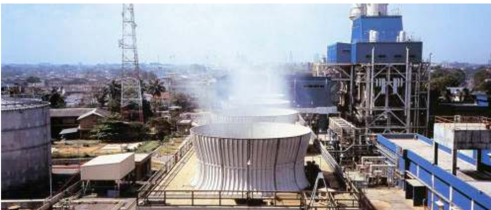
Figure 46: Kelanitissa Power Plant Image Courtesy: lntsnl.com
