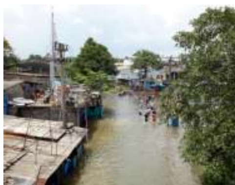
Figure 122: Inundated Colombo – Hanwella Low Level Road near New Kelani Bridge Source: Flood Hazard Assessment & Hydraulic Modelling; deltares, adpc & cecb, 2017
