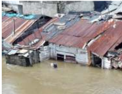
Figure 123: Partially inundated improvised buildings on the left bank of the Kelani River – Closure Look | Source: Flood Hazard Assessment & Hydraulic Modelling; deltares, adpc & cecb, 2017
