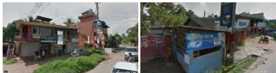
Figure 6.13: Existing situation of Walgama
