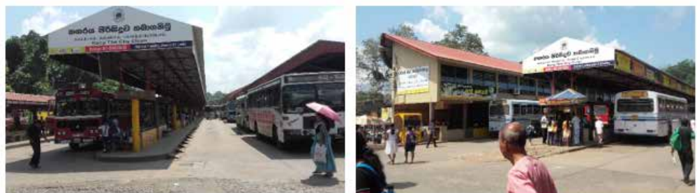
Figure No. 6.3.2.2 : Existing Bus Terminal of Ratnapura Captured by : Hasini Artigala, March 2018
