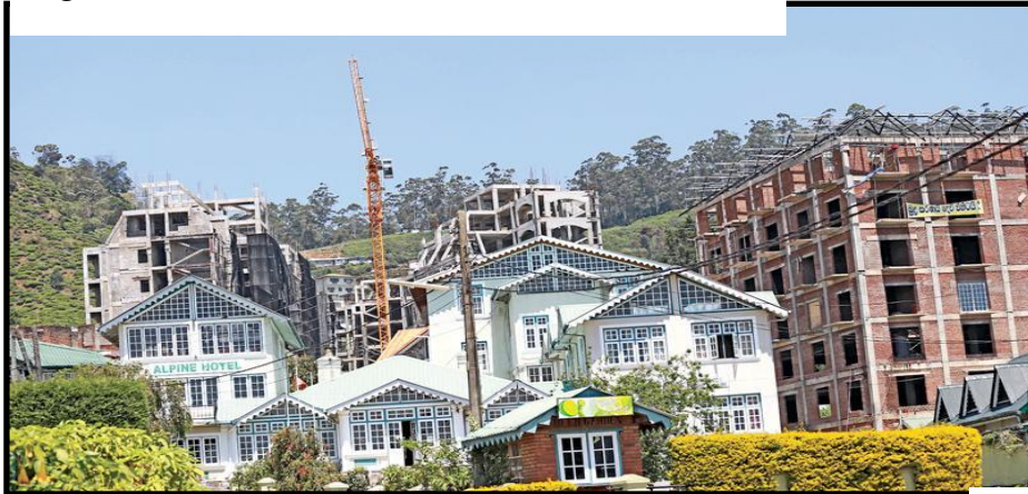
Figure 5.18 New construction covered the Mountain
