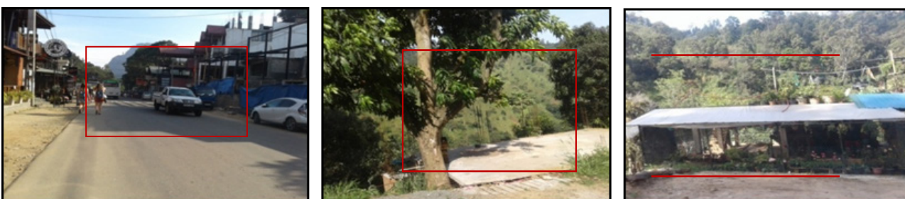
Figure No 5.4: Unauthorized constructions in the Ella Town
