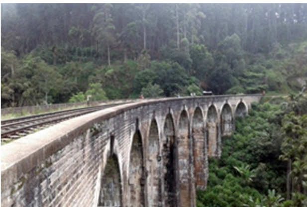
Arches Bridge in Demodara
