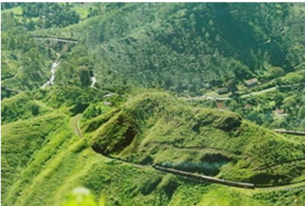
Demodara Rail Track – Engineering Masterpiece
