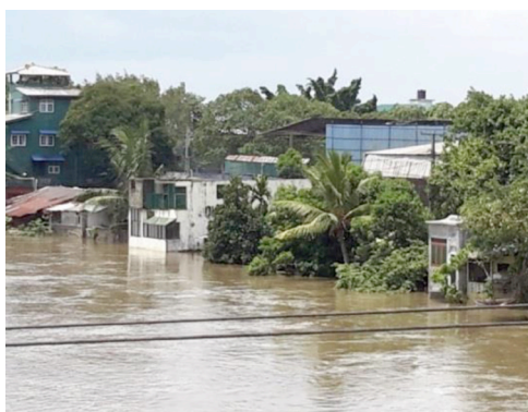
Figure 121: Partially inundated houses on left bank of Kelani River on 20th May 2016 (approx. 2.2m flood water level) Source: Flood Hazard Assessment & Hydraulic Modelling; deltares, adpc & cecb, 2017
