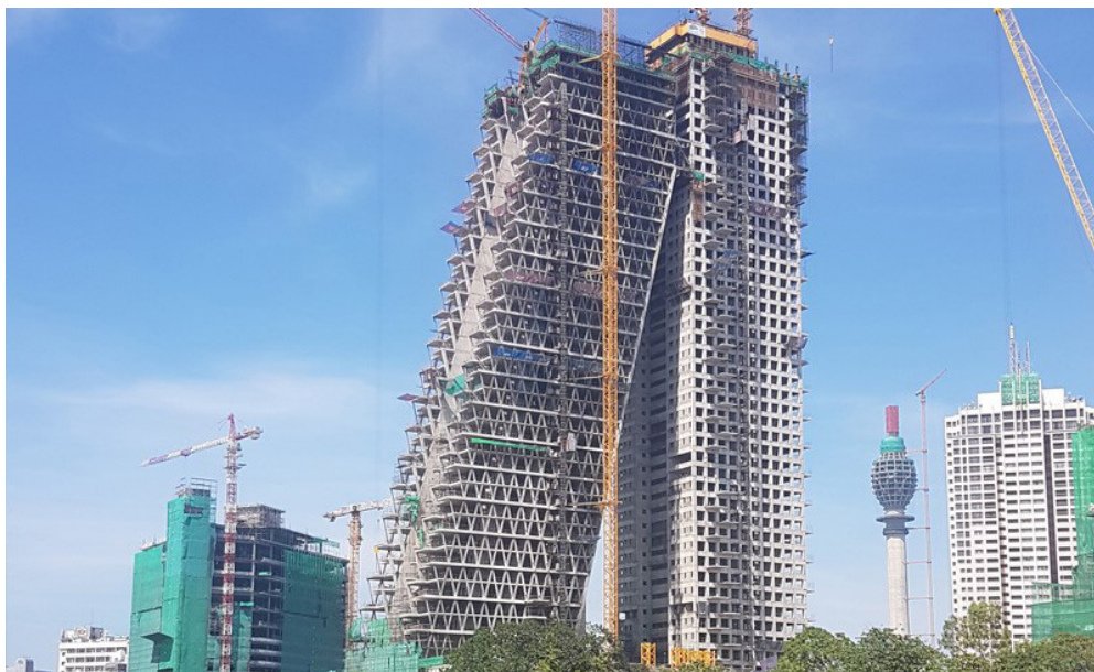
Figure 150: Altair Building (Mixed Development) located at Gangaramaya, Colombo in Construction | Image Courtesy: skyscrapercity.co
