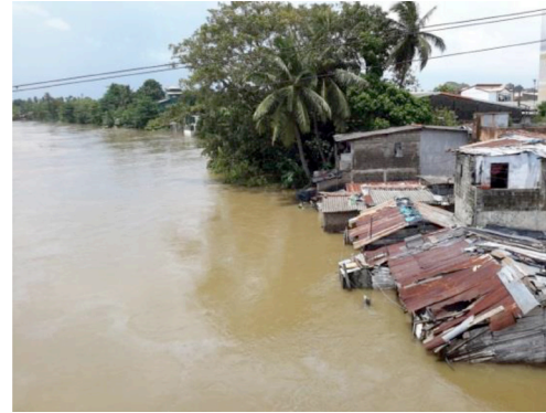
Figure 124: Partially inundated improvised buildings on the left bank of the Kelani River Source: Flood Hazard Assessment & Hydraulic Modelling; deltares, adpc & cecb, 2017
