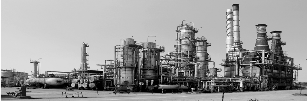
Figure 45: Kolonnawa Petroleum Refinery Image Courtesy: ceypetco.gov.lk
