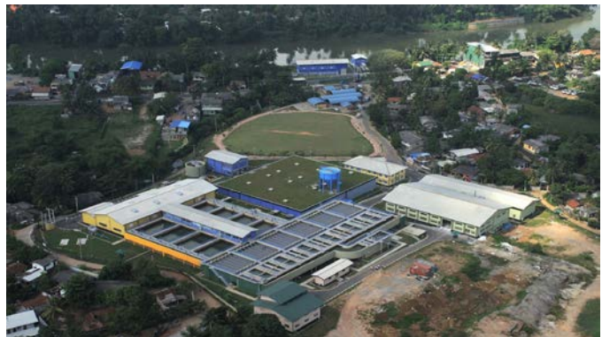
Figure 2. 7 Kelani River Right Bank Water Treatment Plant Source: NWSDB -2018
