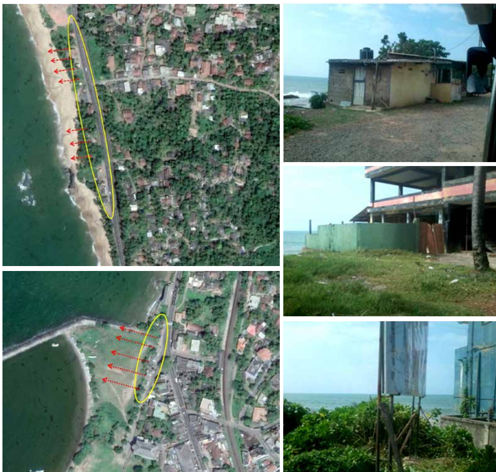
Figure 3.6 : Section of beach line covered due to unauthorized constructions.
