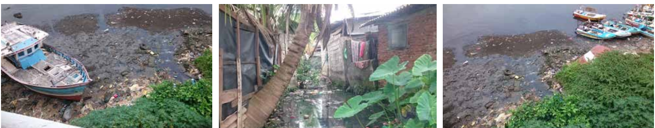
Figure 6.10 : Existing drainage and canal system in Beruwala uc area Source : photography by beruwala planning team, Kalutara district office (2018)
