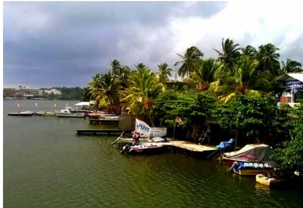
Figure 3.7: Unauthorized constructions in the Benthara river reservation | Source: Photography by Beruwala planning team, Kalutara District Office – 2018
