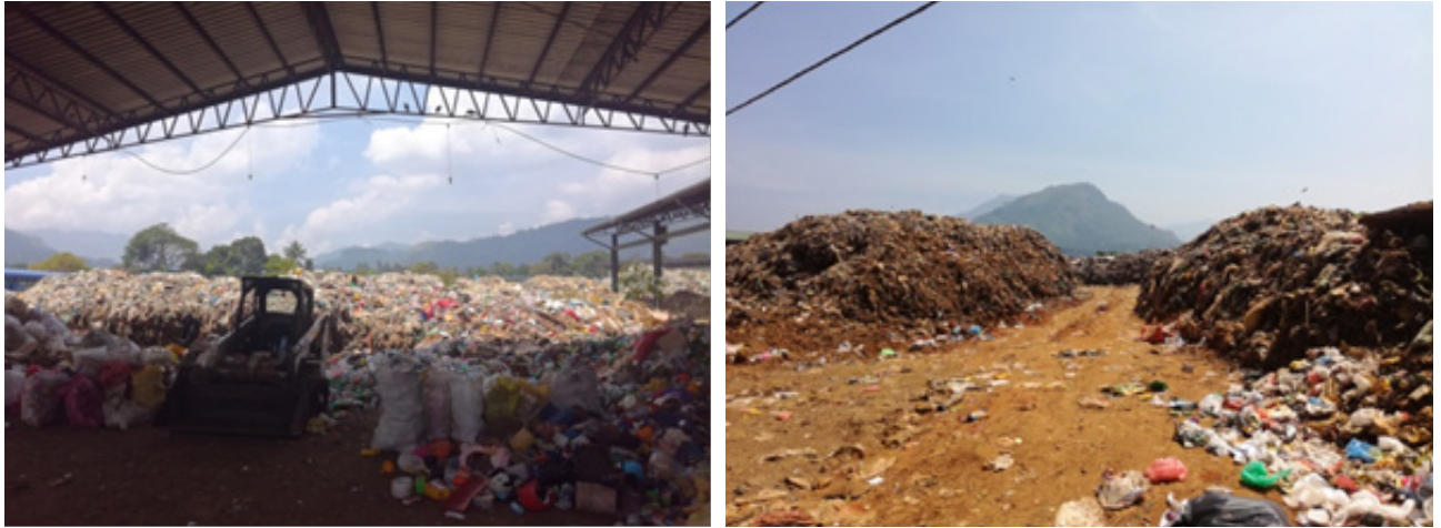
Figure No 5.6: Current Waste Yard
