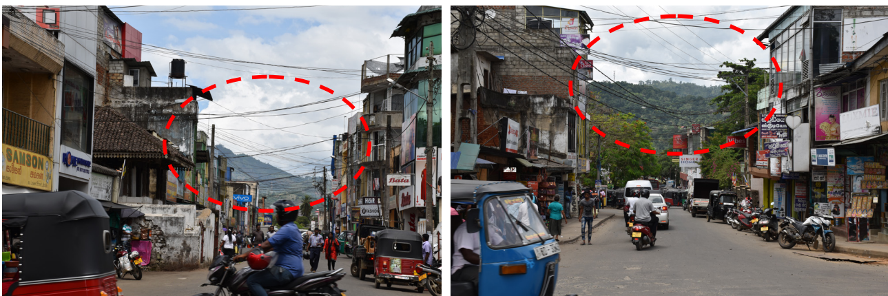
Figure No: 5.10: Improper electricity lines and telecommunication cables
