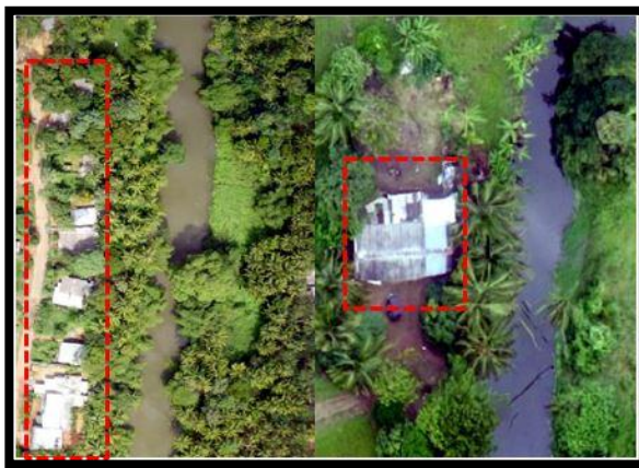
Figure 5. 25 Unauthorised construction in reservation MalwathuOya
