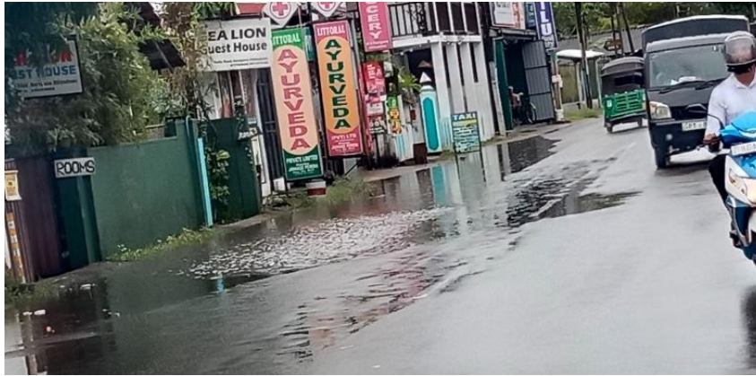
Figure 5.28: Lack of drainage facilities along the Matara –Colombo road near the Hikkaduwa Urban Council Source: Sothern provincial Office, Urban Development Authority
