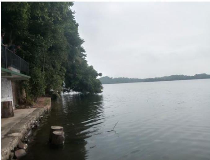
Figure 5.17: Unauthorized constructions in the Rajgama lagoon area
