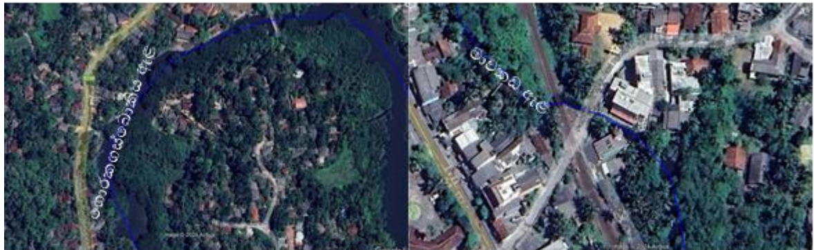
Figure 5.29: Illegal constructions near canal reserves Source: Sothern provincial Office, Urban Development Authority
