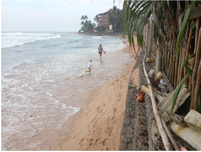
Figure 5.12 : Unauthorized construction of security walls along Hikkaduwa beach
