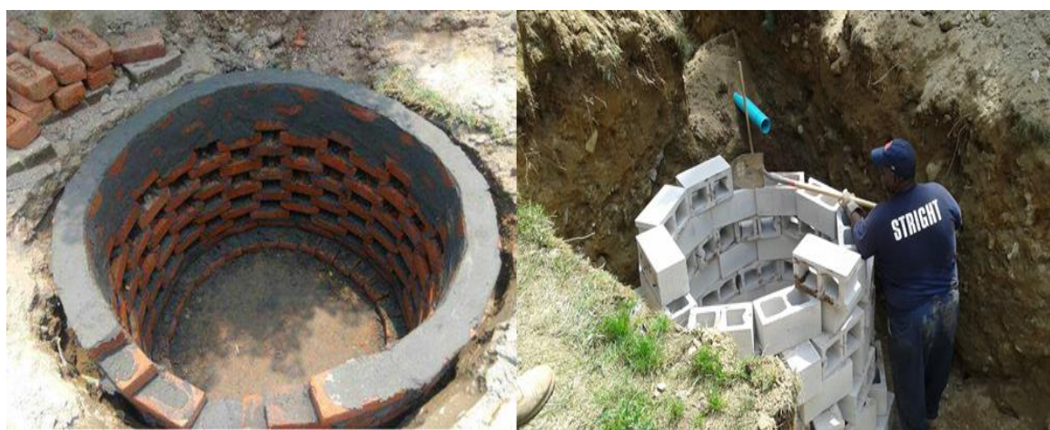
Figure 6.19: Soak Pit System for Kitchen Wastewater Management
