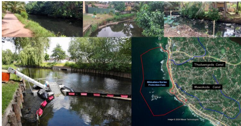
Figure 6.65: Installation of garbage traps in Mawakada and Thuduwegoda canals
