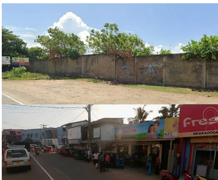
Figure 5.14: Beach view is blocked by the boundary walls Source: Galle District Office, Urban Development Authority
