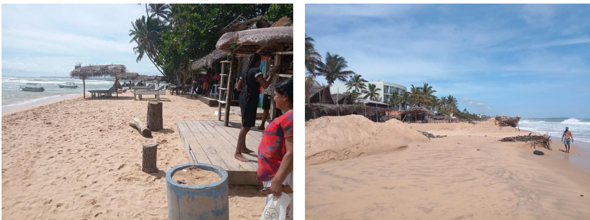
Figure 5.11 : Unauthorized constructions along Hikkaduwa beach
