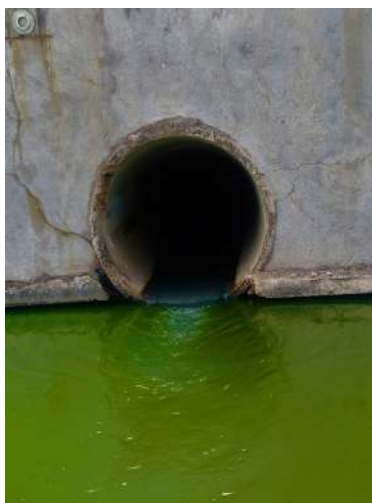
unauthorized sewer and drainage connections continuing the lake pollution
